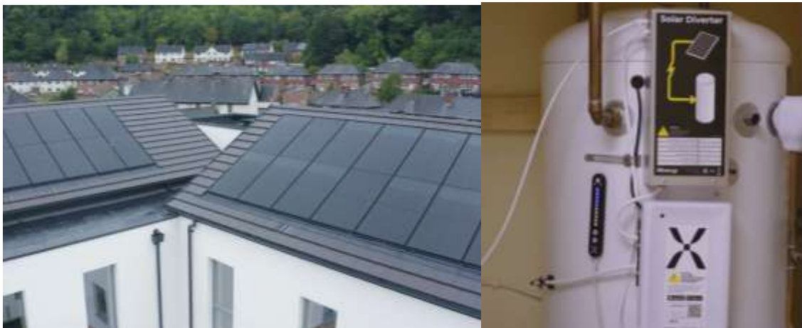
Figure 12. Images from a smart PV hot water solution for 15 new-build flats and 23 existing homes at William Angie Court in Welshpool, Mid-Wales (supplied by Mixergy )
